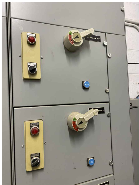
PUMPS P-5 AND P-6 DISCONNECTS IN MCC
