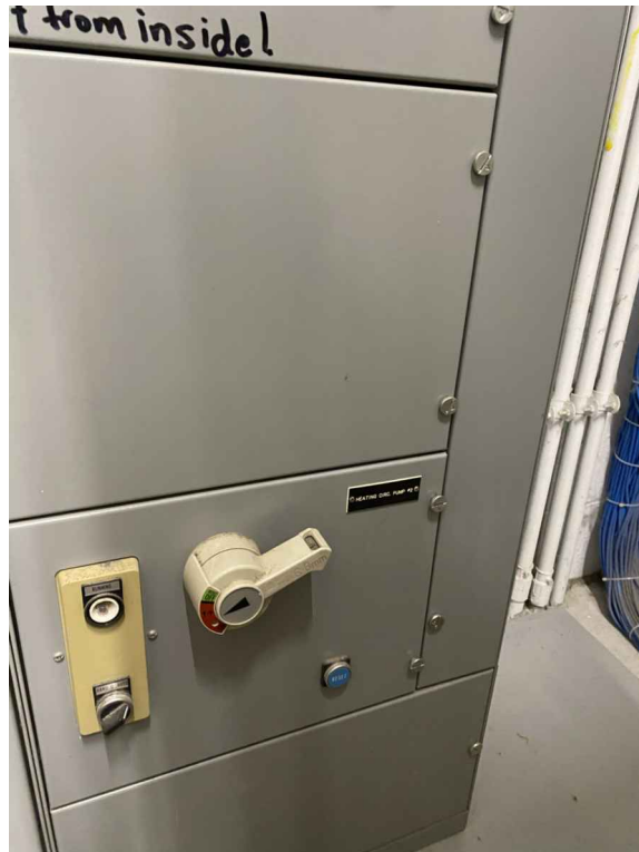
PUMP P-1 DISCONNECT IN MCC
